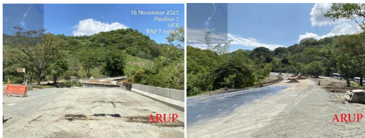
Figure 3. K92.9 Bridge 3 status as of November 16th, 2023
